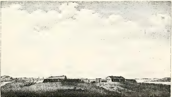
A Front View of the Lines taken from the advanced Post near Brown's House.
